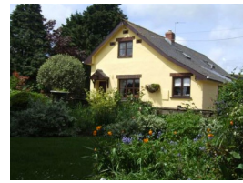
Barn Cottage & Stable Cottage
